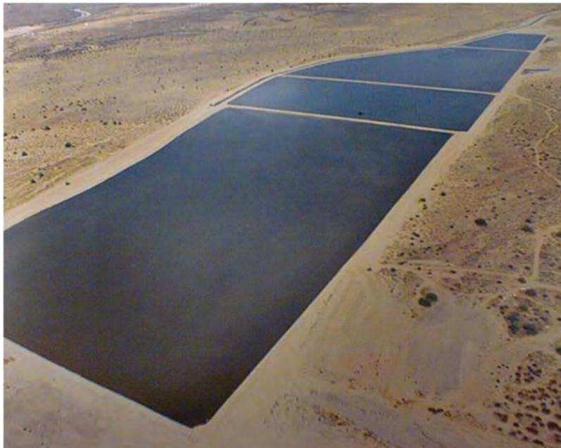
Spreading basins, such as the Granite Reef Underground Storage Project above, allow water to percolate into the soil and are used to recharge the groundwater tables.
