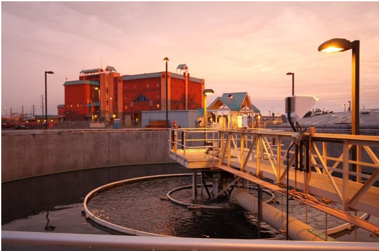
A surface water treatment plant. Source: City of Phoenix Water Services Department.
